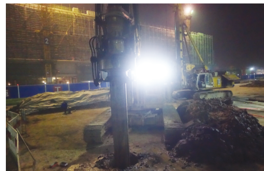
临泉路与四里河路交口工地仍在施工
